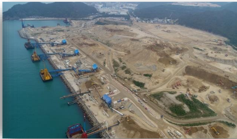
本地填海工程於將軍澳第137區填料庫利用運輸帶提取公眾填料 Collection of Public Fill from the Tseung Kwan O Area 137 Fill Bank by local reclamation projects via conveyor belts
