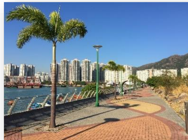
屯門綠化總綱圖(青山灣海濱長廊) Greening Master Plan for Tuen Mun (Castle Peak Bay Waterfront Promenade)
