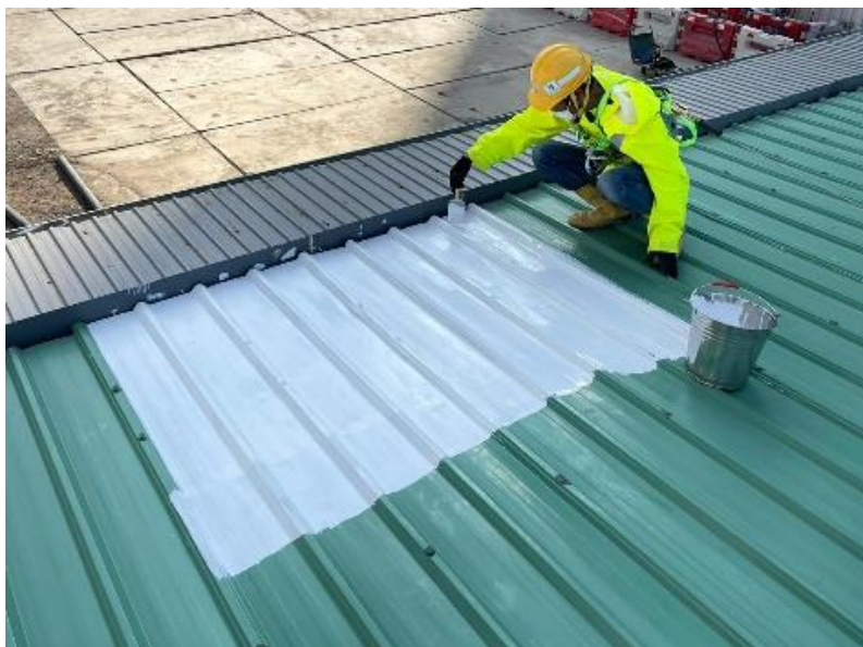
於地盤辦公室應用被動式輻射製冷塗層 Adoption of passive radiative cooling paint at the roof of site office
