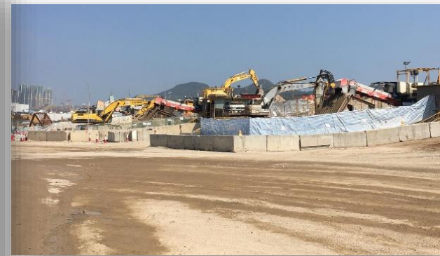
破碎混凝土及石塊可循環再造成200級再造石填料 Recycling of broken concrete and rock pieces into Grade 200 recycled rockfills
