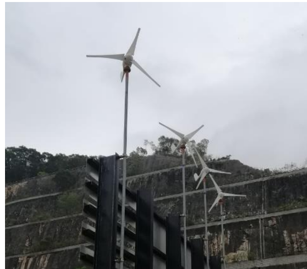
於地盤採用風力發電機 Installation of wind turbine at works area
